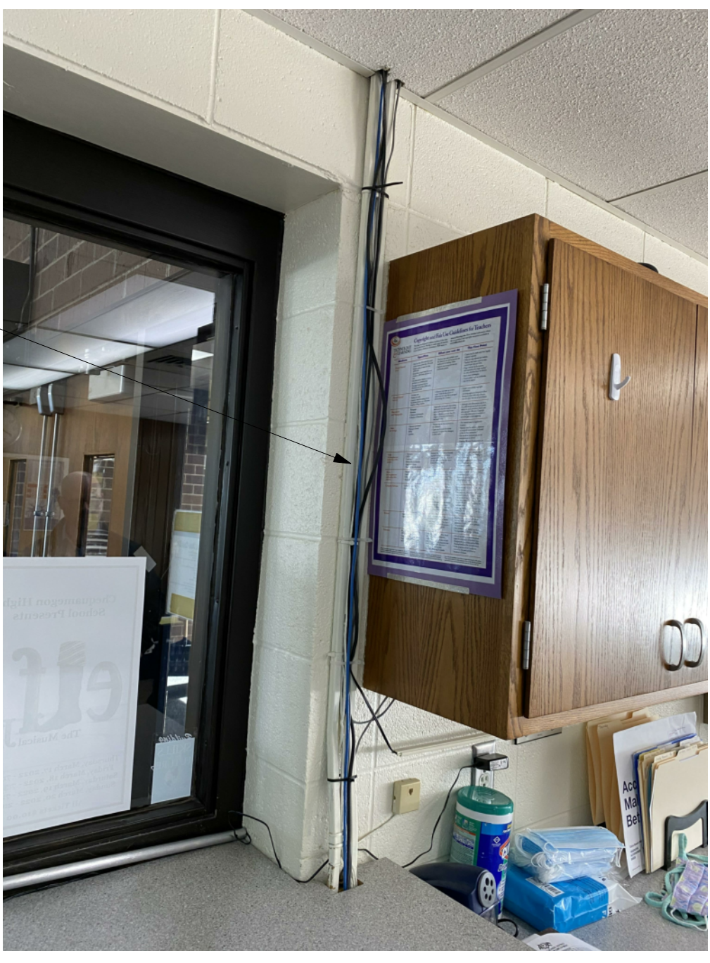
Remove surface raceways, data cables and coaxial cables, verify use of cables and reinstall if still required, provide new lengths of cables back to source.
